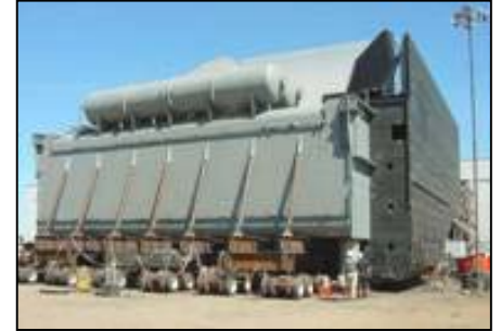
Spillway Weirs – the ‘Fish Slide’
